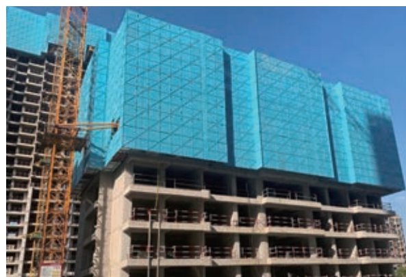
脚手架覆网 Scaffold Coverings
